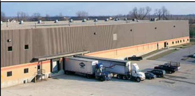
Link-Belt Parts Distribution Center
